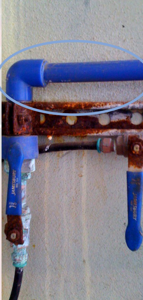
Air-Pro® at a bleach plant without corrosion.
