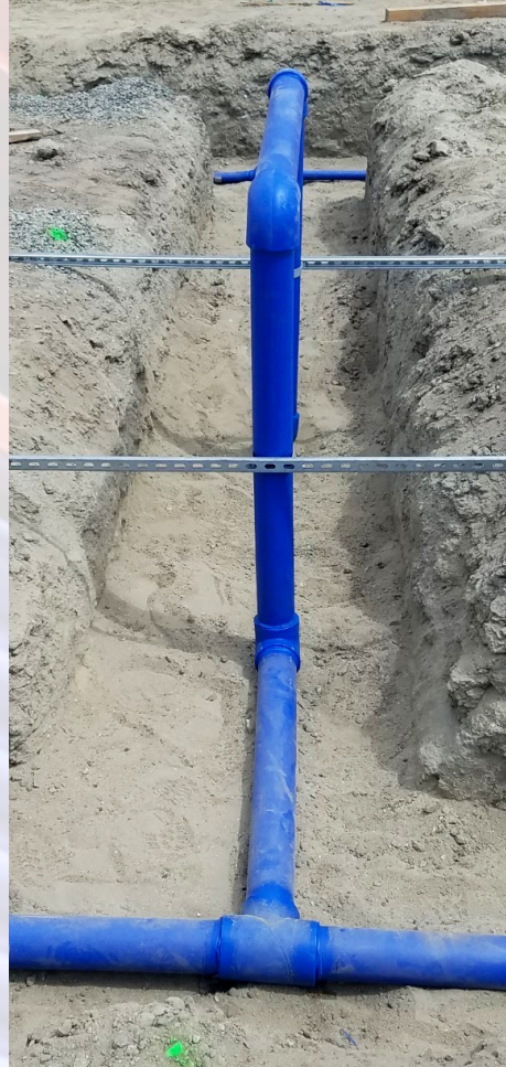
Air-Pro® in a buried application.
